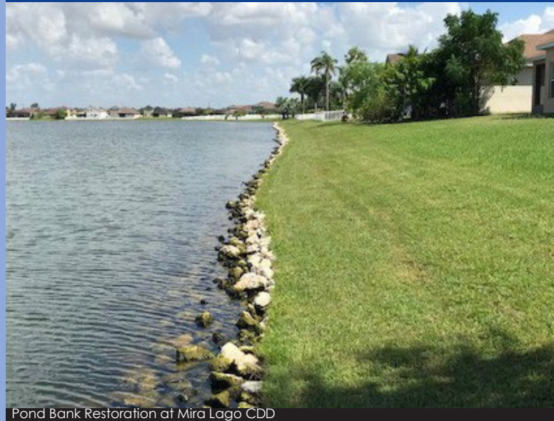
Pond Bank Restoration at Mira Lago CDD
