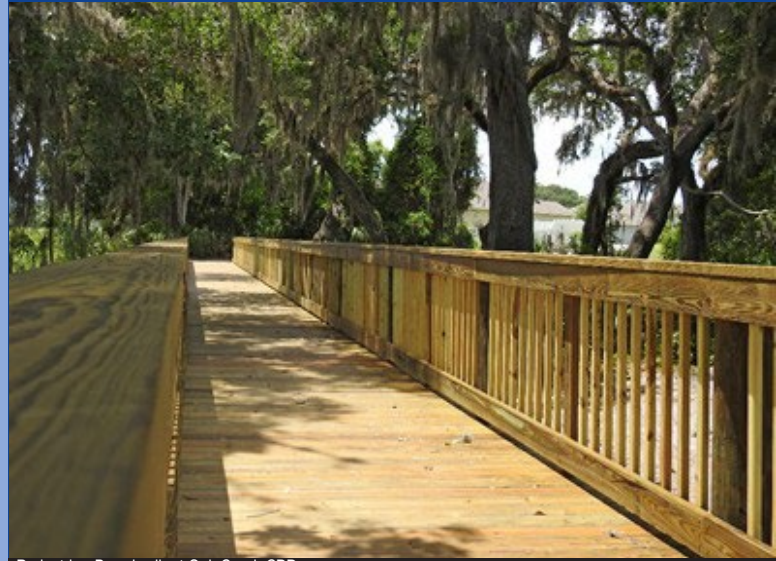
Pedestrian Boardwalk at Oak Creek CDD
