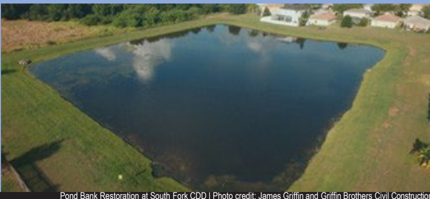
Pond Bank Restoration at South Fork CDD | Photo credit: James Griffin and Griffin Brothers Civil Construction
