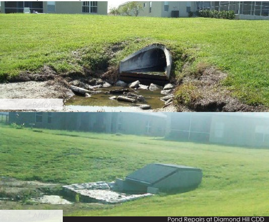
Pond Repairs at Diamond Hill CDD
