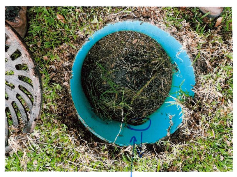
drain Pipe connection hole.
