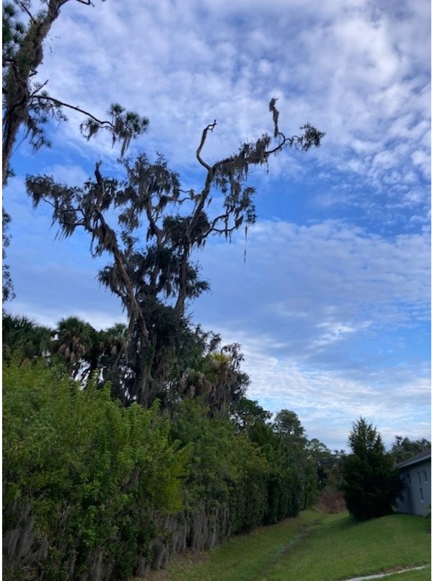
Utilize Crane already on site to cut and remove two large dead laterals
